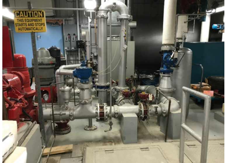
Eabametoong First Nation Water Treatment Plant
