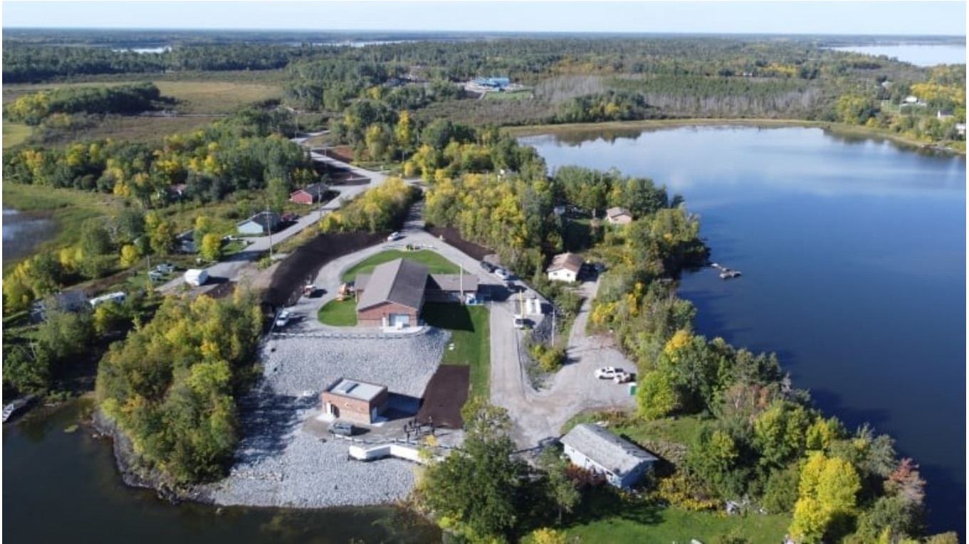
An aerial view of the award-winning new water treatment facility in Shoal Lake 40 First Nation in Northwestern Ontario. (Tyson Koschik/CBC)
